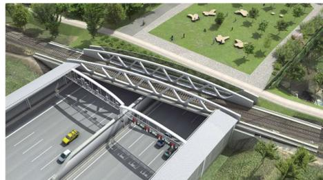
on the tunnel roof. The roof to the tunnel will be in prestressed concrete because of the long spans and the later usage. This will be the first time that such spans and this type of construction with a prestressed roof slab have been used in Germany on this scale. The City of Hamburg will be holding a design competition for the landscaping to the tunnel roof.
